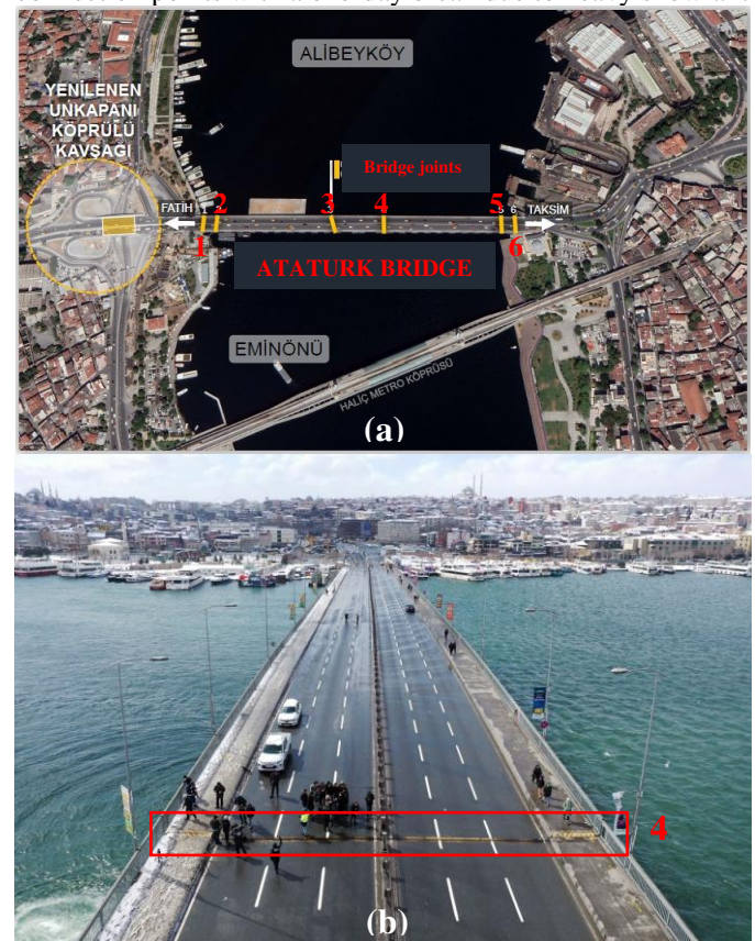
Figure 1. Atatürk Bridge (a) location (b) gap in the deck.
