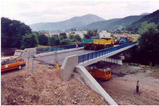
Figure 7: Loading of a bearing
