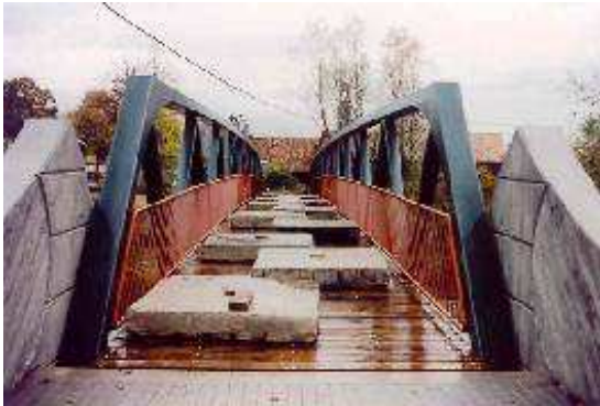
Figure 3: Static tests on a footbridge.
