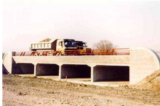
Figure 10: Central loading of a multiple span frame
