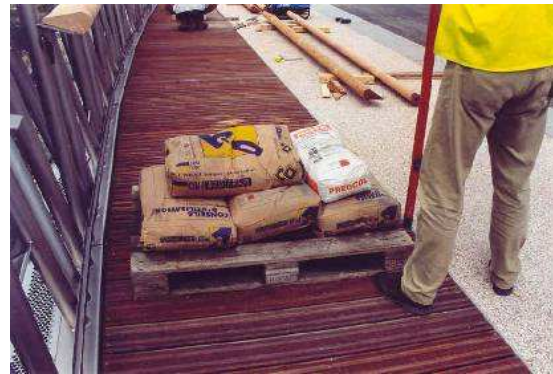
Figure 2: Placing a load on a pavement.
