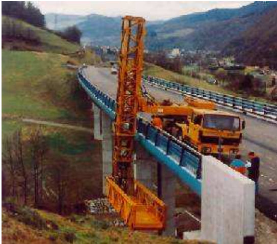
Figure 5: Inspection using a temporary gangway
