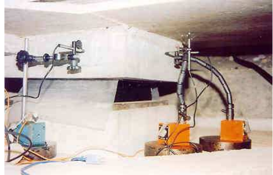
Figure 4: Sensors for measuring displacements on a bridge bearing.
