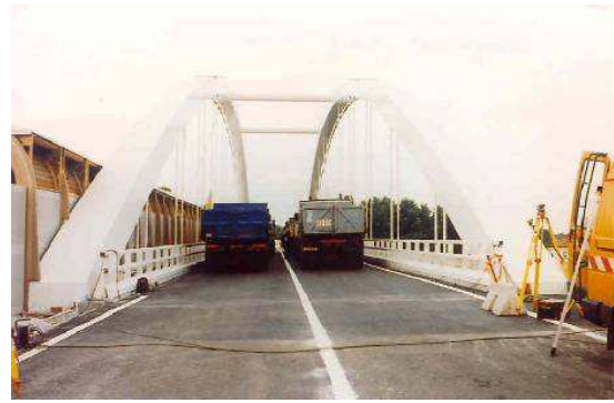
Figure 13: Measurement of deflections during tests on a bow string.
