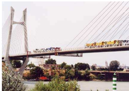
Figure 11: Test loads on a cable-stayed bridge
