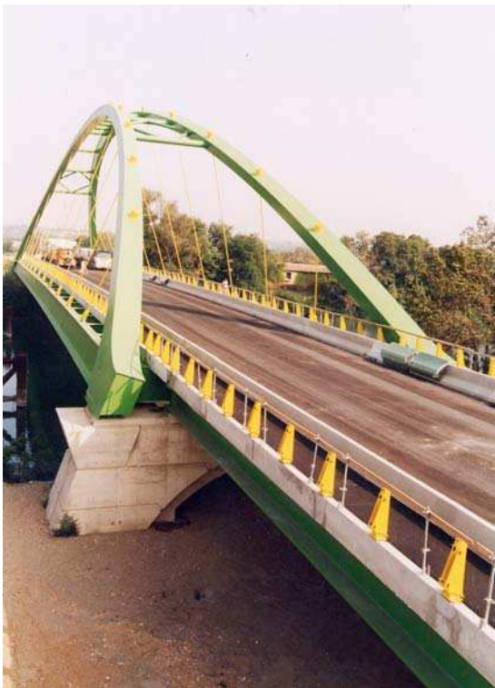
Figure 9: Loading test on a bow-string bridge
