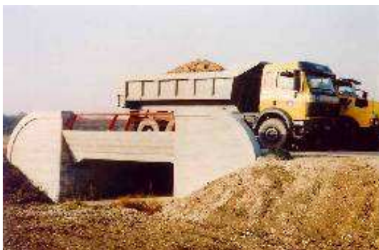
Figure 8: Loading test on a short span bridge
