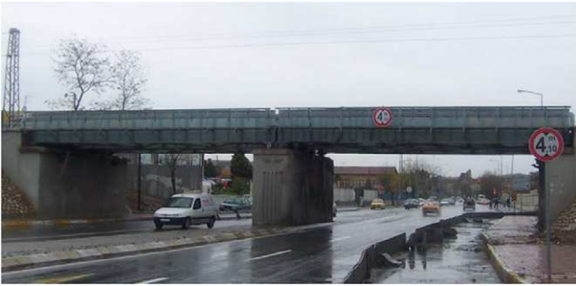
Fig. 1. A general view of the bridge.
