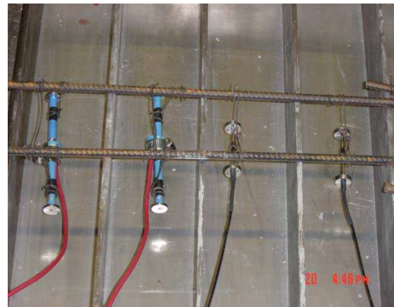
Fig. 8. Sensors suspended in creep and shrinkage forms
