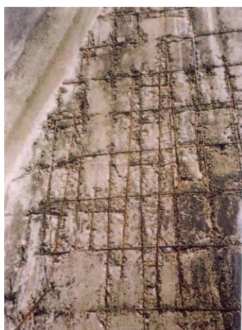
Fig. 9 Cooling tower mantle
