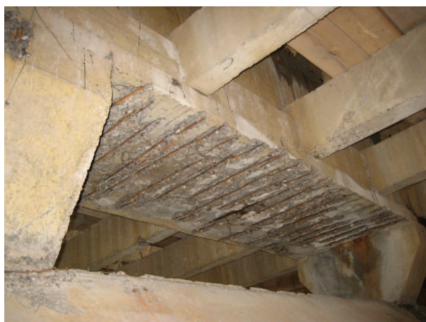
Fig. 10 Beam for sprinkler installation
