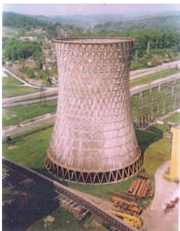
Fig. 11 Cooling tower, Thermoelectric Power Plant in Tuzla
