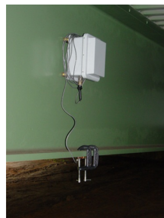
Figure 1. ISBMS mounted on girder
