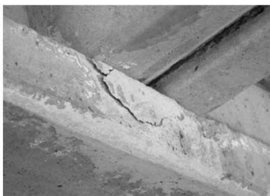
Figure 18: Insufficient concrete cover and stirrups corrosion in the beam
