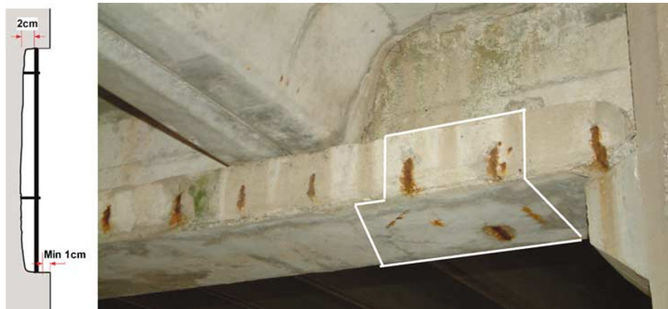
Figure 39: Forming of opening in concrete at the place of corroded rods
