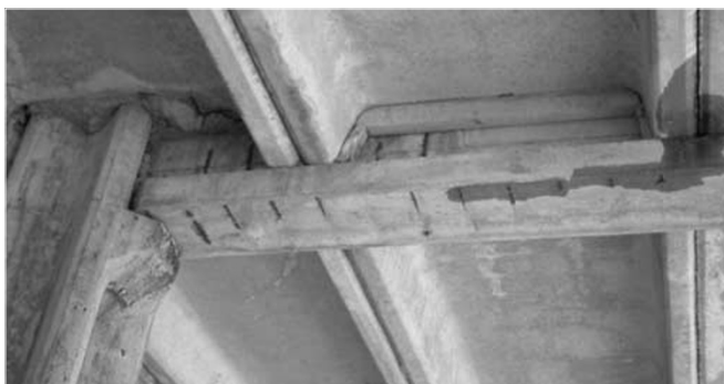
Figure 18: Insufficient concrete cover and stirrups corrosion in the beam
