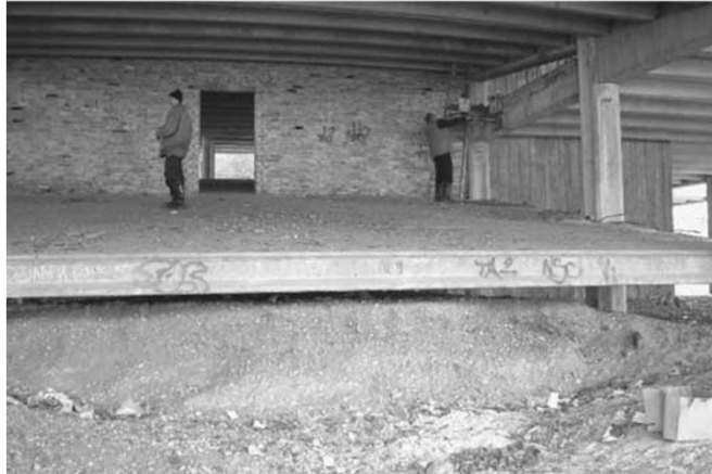
Figure 6: Uncompleted section of approach ramp
